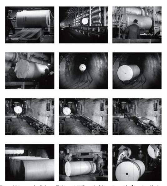
Paper delivery to the Chicago Tribune: 1–2 Paper is delivered straight from the ship into a warehouse; 2–9 Reams of paper are then loaded onto a dolley; 4–7 The dolley travels on to Tribune Tower on train tracks in an underground tunnel before being unloaded onto a ramp at the other end by a mechanical tipping device; 8 The empty trolley returns to the warehouse automatically; 10–12 Reams of paper are then lifted up to the press room and taken to the presses.
